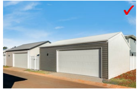
Garages and sheds on lanes have coordinated materials.
