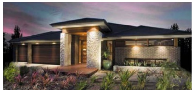
Figure 10: This design incorporates wide eaves (5.5), stone and timber elements (5.2), a translucent porch (5.2) and a third garage discreetly set back from the main garage door (5.3)
