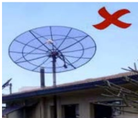
Satellite dish above roof
