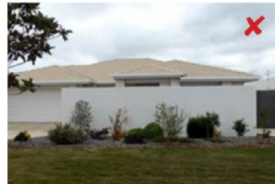
Solid fencing forward of building
