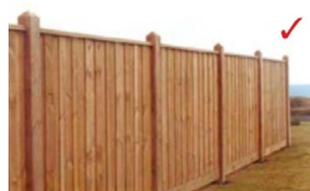
Lapped and Capped (corner blocks)
