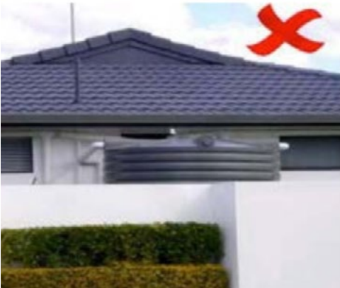
Rainwater tanks visible
