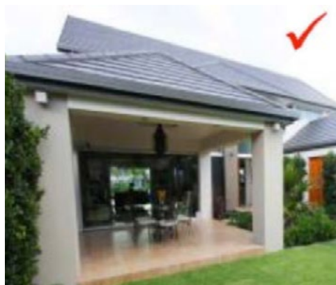
Verandah construction matches house
